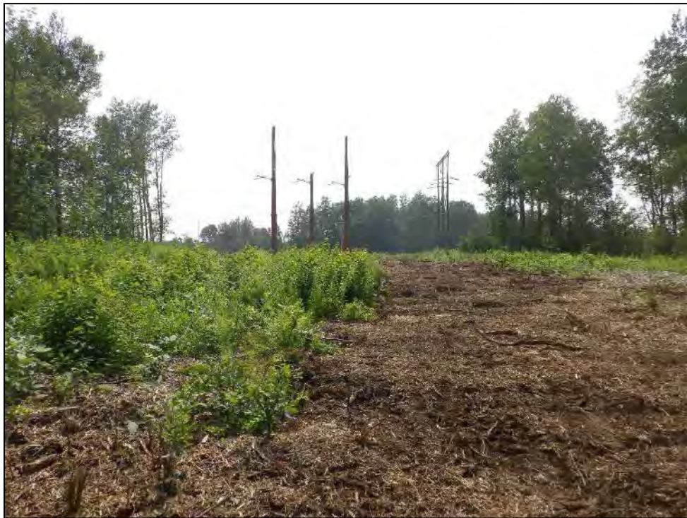
Figure 39: View facing west within the survey area (disturbed-construction) (R0016616).
