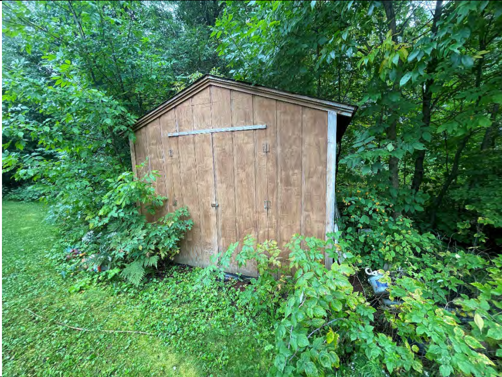
Photograph 5 September 11, 2025 Direction: South Subject: Shed (3635)
