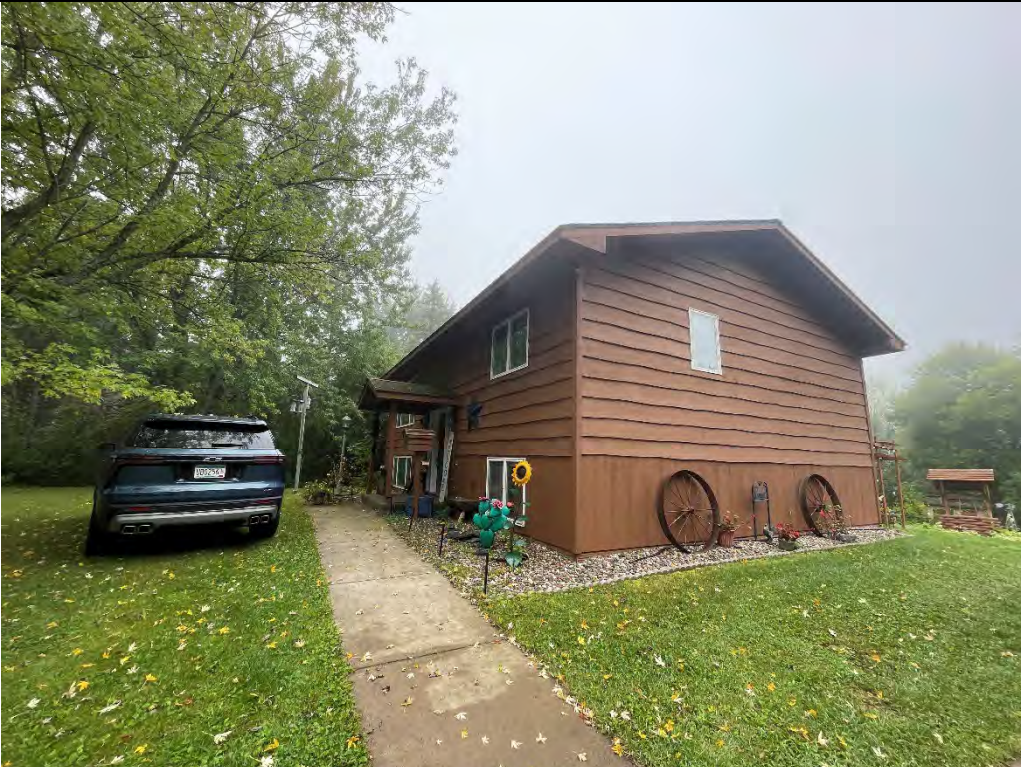
Photograph 2 September 11, 2025 Direction: Southwest Subject: House (3635)
