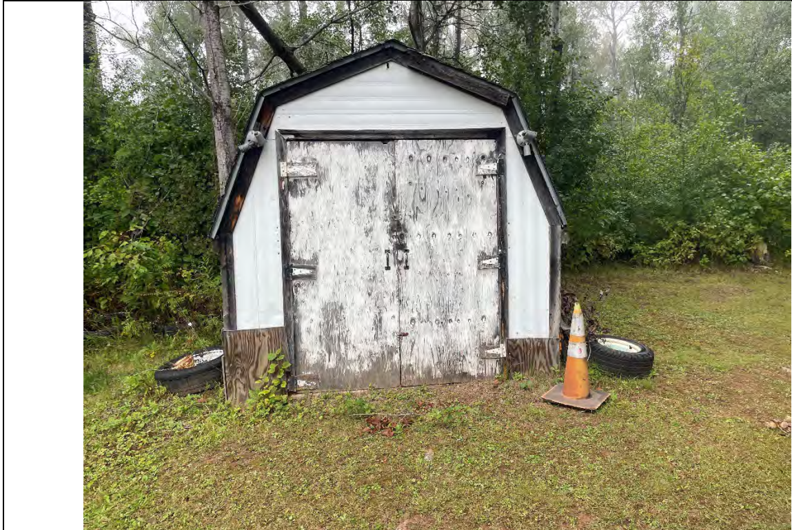
Photograph 13 September 11, 2025 Direction: North Subject: Shed (3589)
