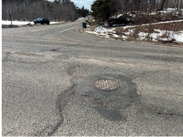
Example of utility casting conditions
